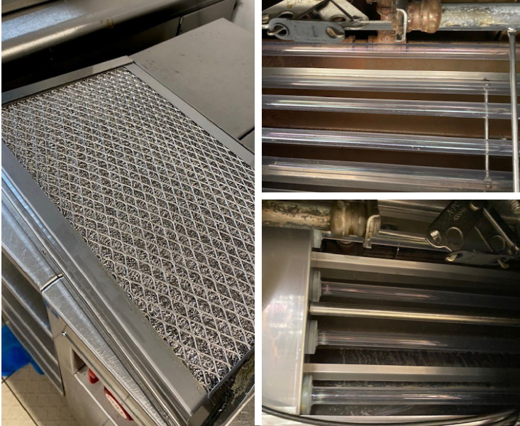
Fryer 1 and 2 - UV-C Lamps and exhaust filter
