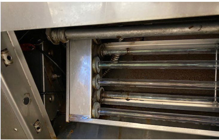
Fryer 1 and 2 - UV-C Lamps and exhaust filter
